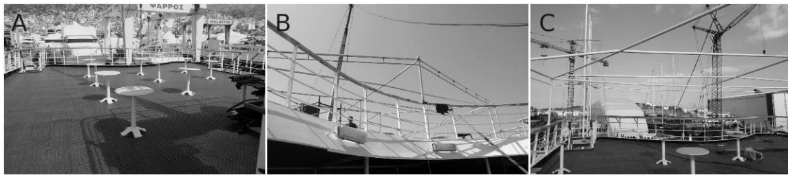
Figure 9a, b, c. Upper Deck Back Side Rail, Existing Situation. Source: Siniša Prvanov
