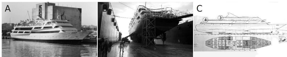
Figure 1a, b, c. m/v John P, Pireus Port (1994), m/v Anna Maru at the shipyard (2016), Section and plan drawing with indicated renovation areas. Source: Hydraiki Naval Company. Greece
