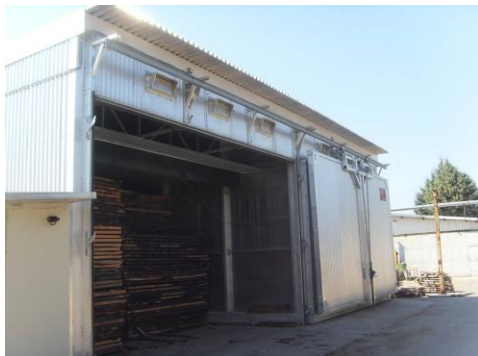
Figure 1. Industrial dry kiln
