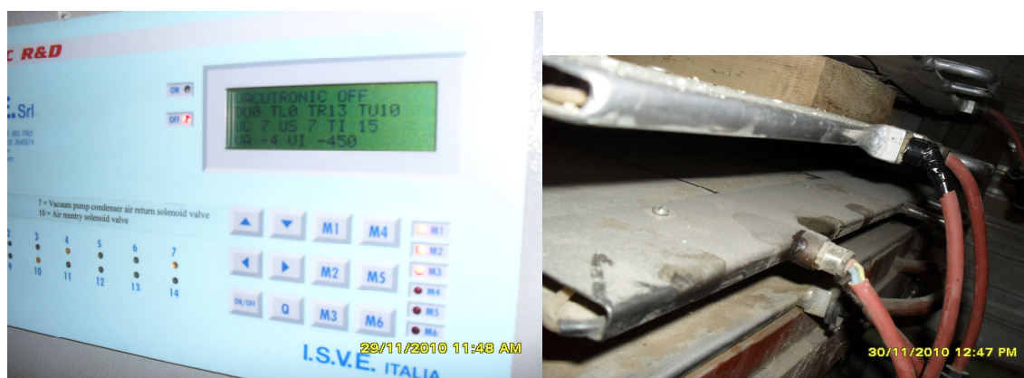
Fig. 5: Control and heating unit of drying
