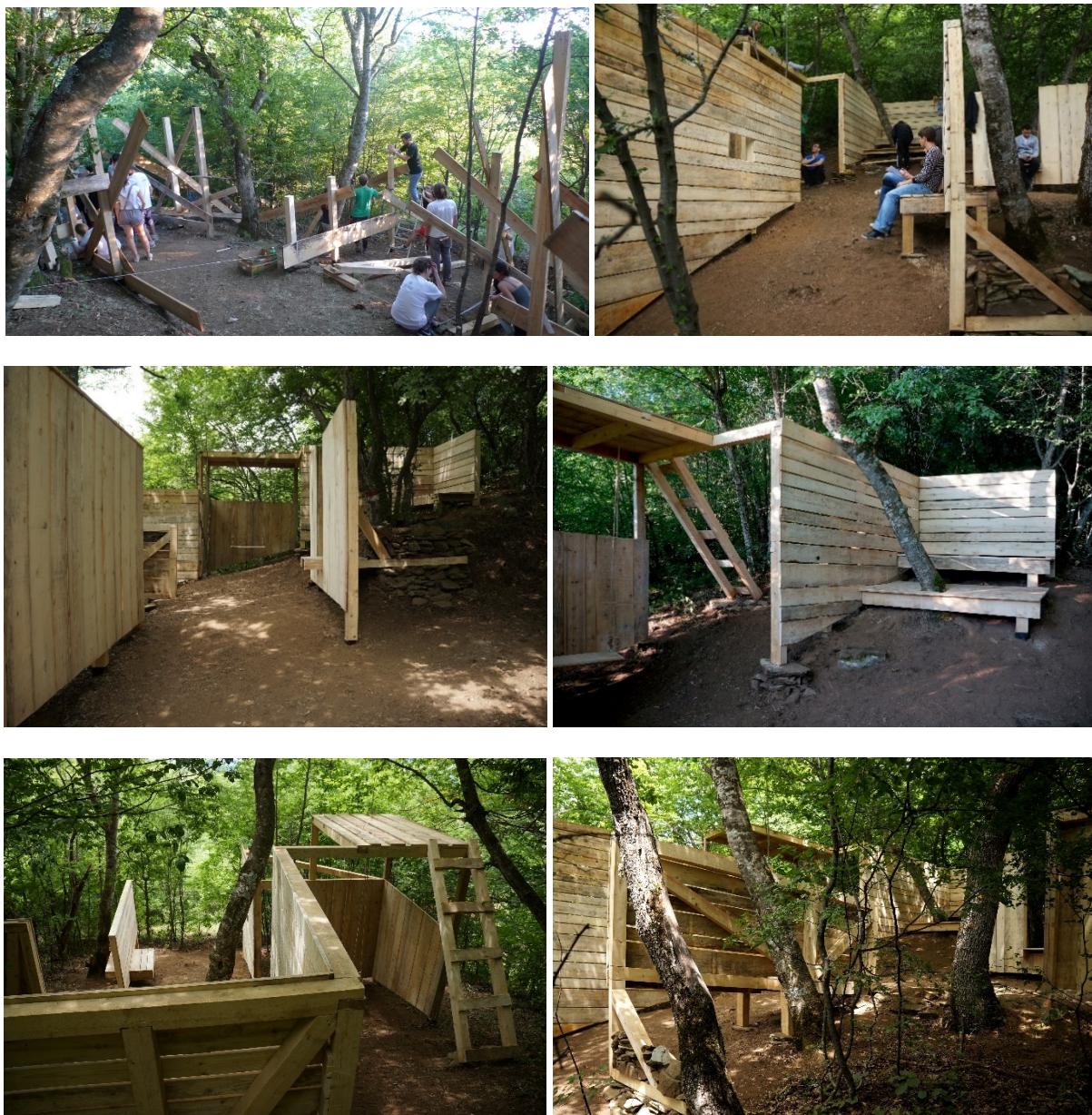
Figure 3. Chapel for Nature, the timber pavilion in the process of construction and finished
