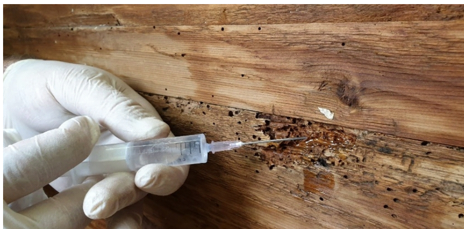
Figure 15. Injection of consolidant
